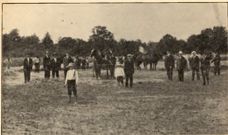
BREAKING GROUND FOR GIRLS' DORMITORY
