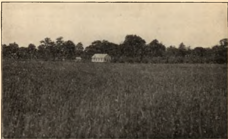
FIRST PRIMARY SCHOOL BUILDING
