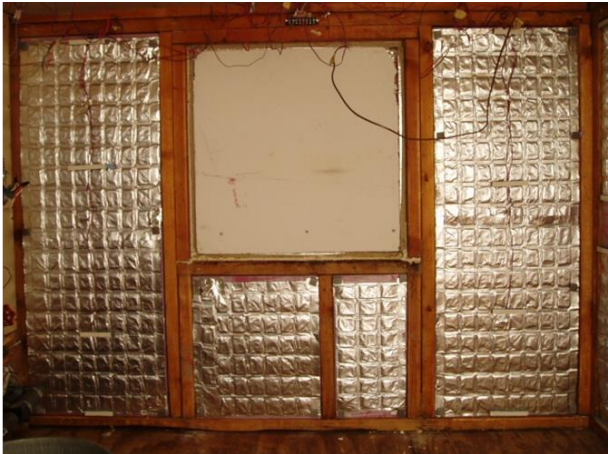
Figure 5: PCM pouches incorporation [26]
